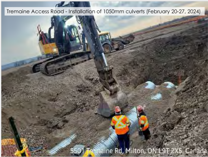
Photo 5: Tremaine Access Road Culvert construction.
